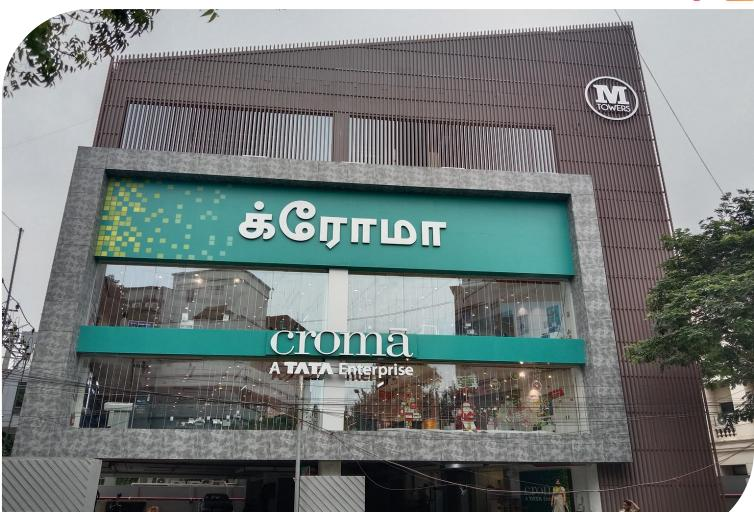
Client: CROMA, Location: TTK Road, Alwarpet. Scope of Work: HPL Cladding, Toughened Glass & Louver Fins
